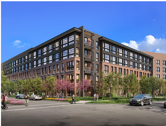
The Laura, a multifamily project at Midway's East River development in Houston, will total 360 units.
